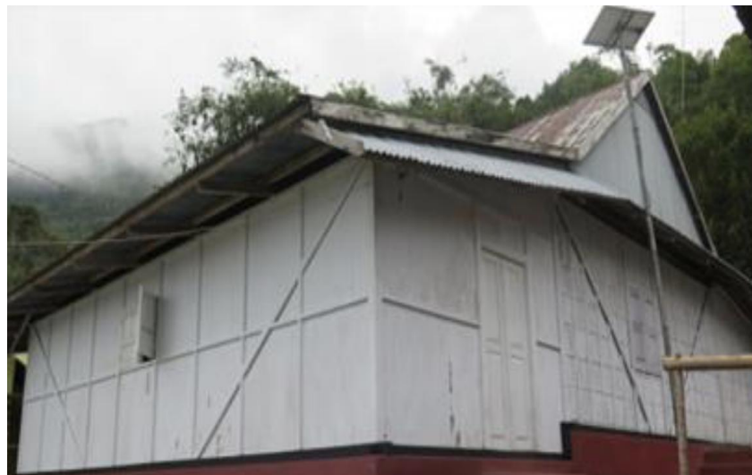
Figure 3. Sowohi Mahifa Traditional House
